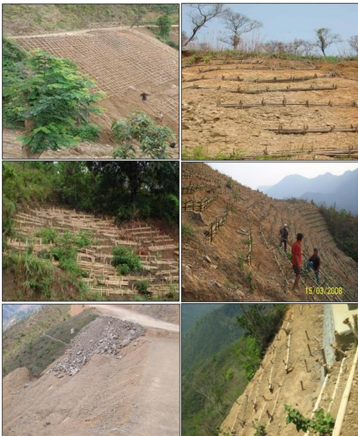
Plate 2: Different measures of bio-engineering in the project road
