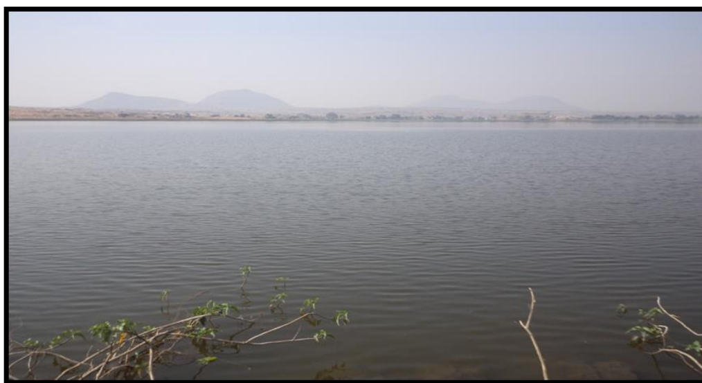
Plate-1: Dedargaon dam
